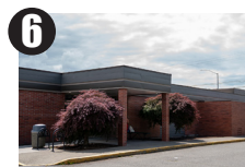
South Tacoma Library 3411 South 56th Street
