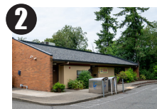
Kobetich Library 212 Browns Point Blvd NE
